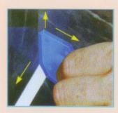
When sealing the corners hold the tool at 45° angle and pull away from the corner (see arrows). Always keep the tool wet to prevent any excess sealer from sticking.
